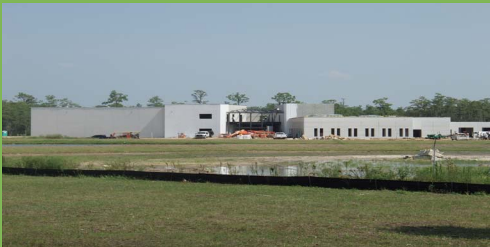
Actual Construction Photo as of 9/12/2007
